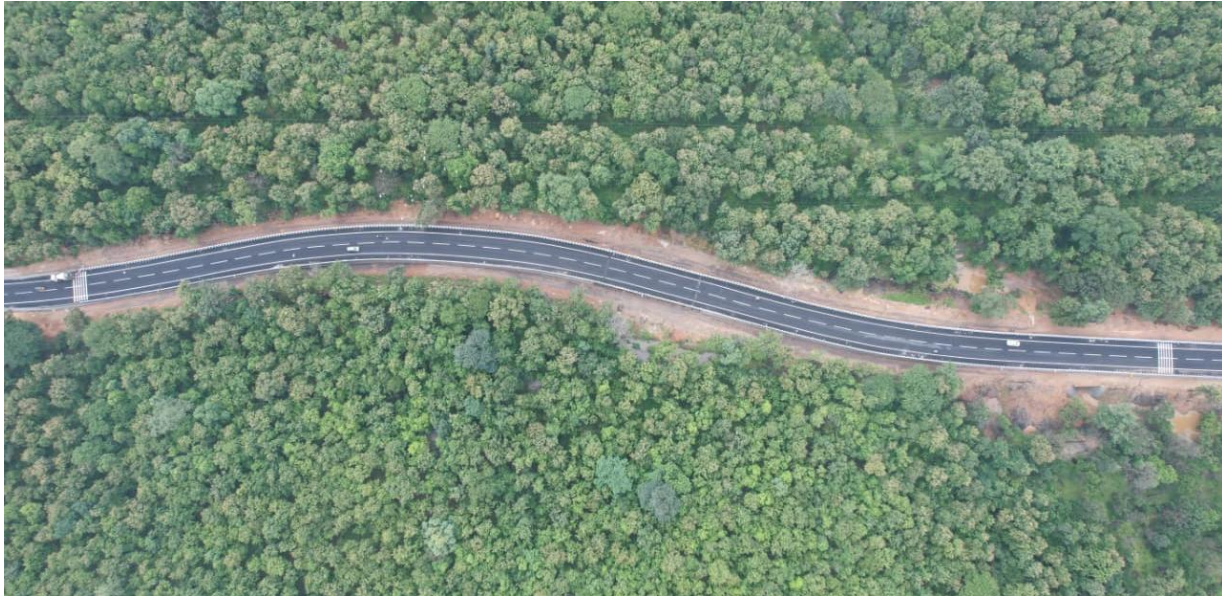
2. Animal Underpass -Nirmal-Khanapur section of NH-61
